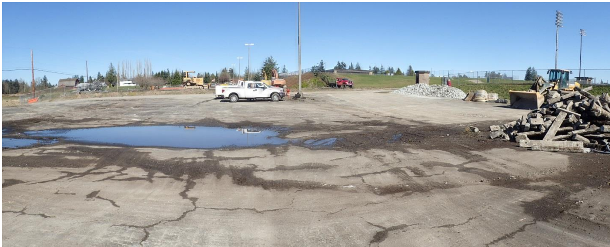
South end of south parking lot; curbs removed
