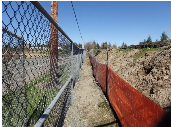
Silt fence along chain link fence at 11 th Ave
