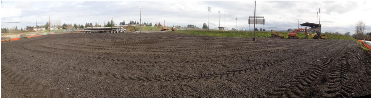
Panorama View from SW corner of southern-most parking area (future water-quality pond)
