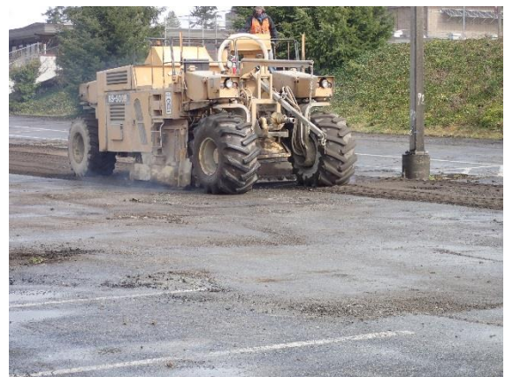
Pavement grinder in operation
