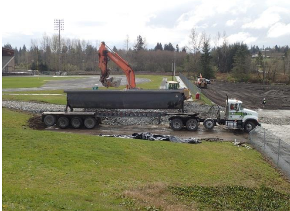
Recycled concrete delivery
